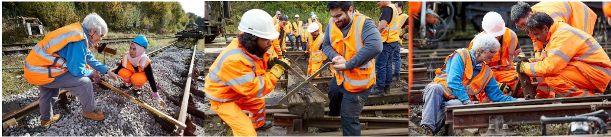
Figure 1. Images of work being undertaken by students.
